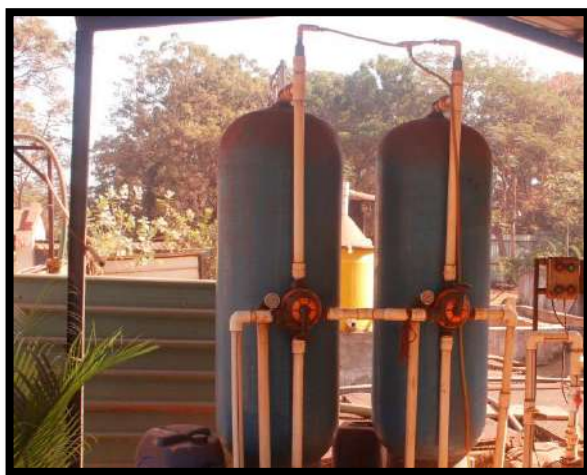
Photo Showing Sewage Treatment Plant installed at Employees base camp
